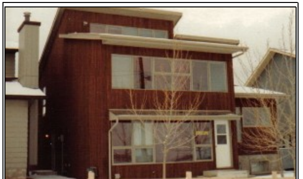
Fig. 13: home for Engineered Homes, builder 1981
