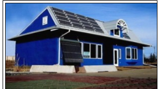
Fig. 21: Energy Plus Eco Office Building, 2002
